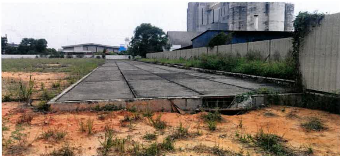
UNDERGROUD ON-SITE DETENTION (OSD) TANK
