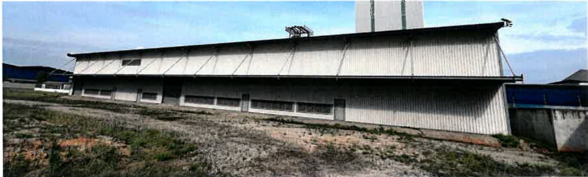
GENERAL VIEW OF THE 2-STOREY MAINTENANCE AND STORAGE WORKSHOP
