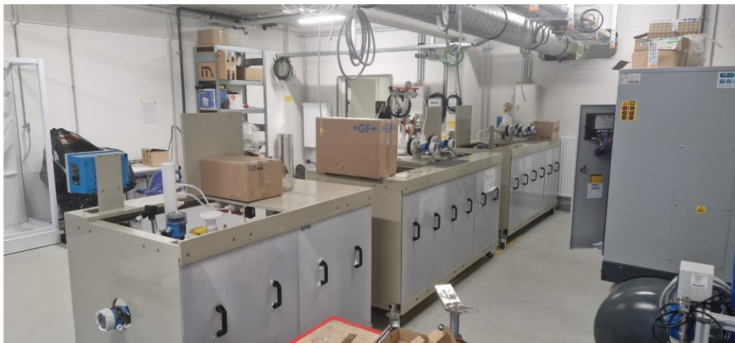
Figure 3 – Pilot Plant Test Equipment
